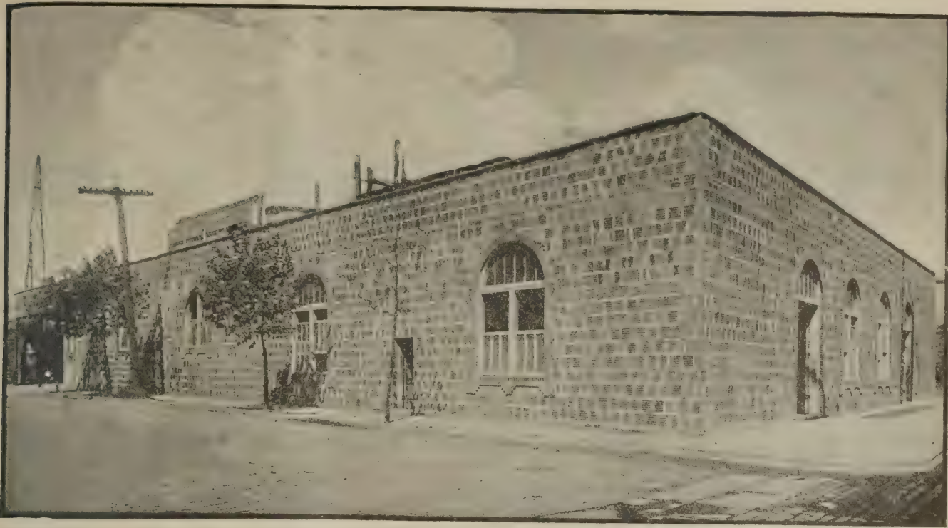
An ice plant of Hollow Tile ready for the stucco finish
